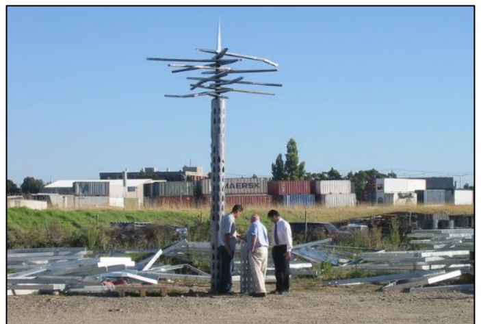
Creation of the steel sculptures off site March 2002
